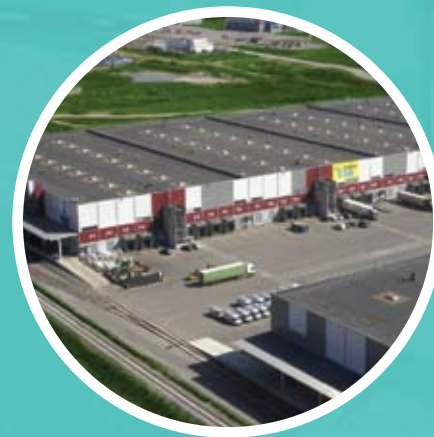
Industrial park "GREENSTATE" 112 ha
