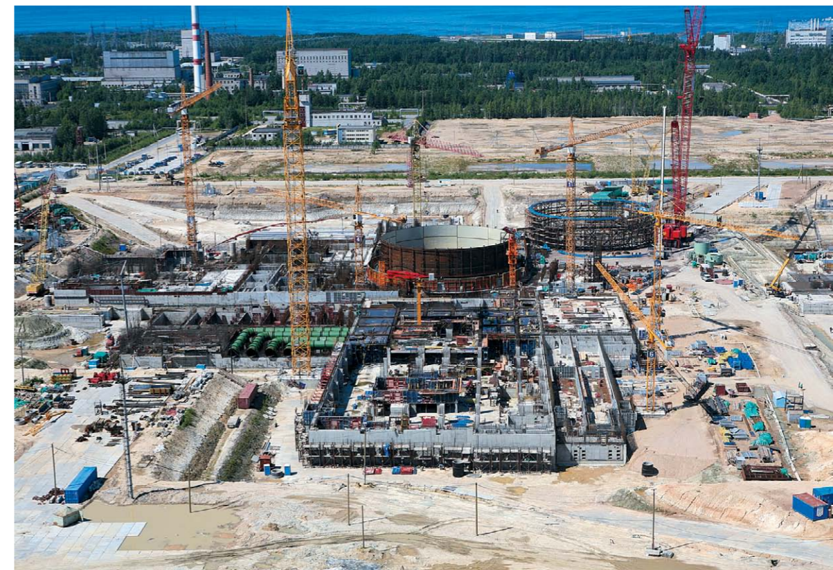
Construction of LAES new buildings
